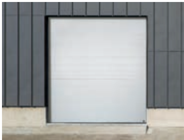
REPAIRED DOOR WITH AMARR 2747 REPLACEMENT SECTION
